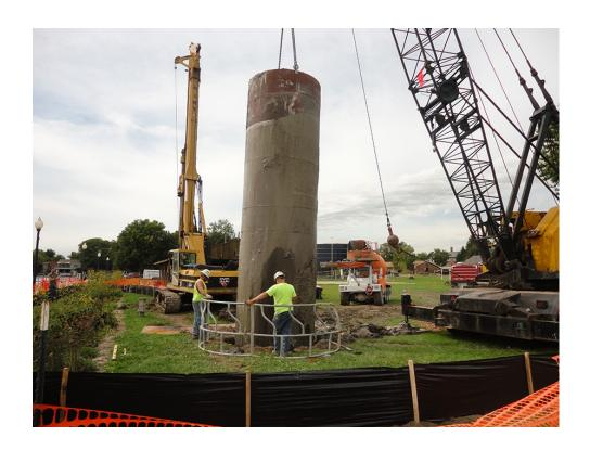
Nearly 80 tons of concrete were used to construct a base that is nearly 7 feet in diameter and 30 feet deep! Such a monumental base is required because, at 160 feet, this flag pole is the tallest in the State of Michigan!
